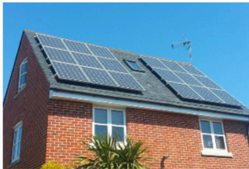
Solar PV Systems & Biomass Heating
