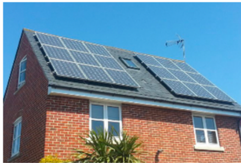
Solar PV Systems & Biomass Heating
